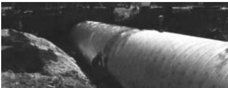
Ease of installation of CSP through existing concrete box.
