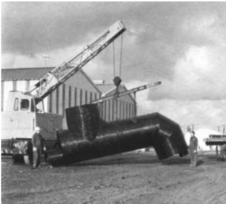
Combination increaser, manhole and elbow in one length of pipe.
