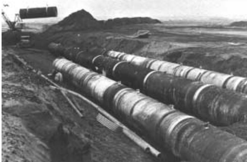
3000 mm (120 in.) diameter, 75 x 25 mm (3 x 1 in.) prefile full bituminous coated and full paved; 1500 m (5000 ft) installed as stream enclosure for runway extension.
