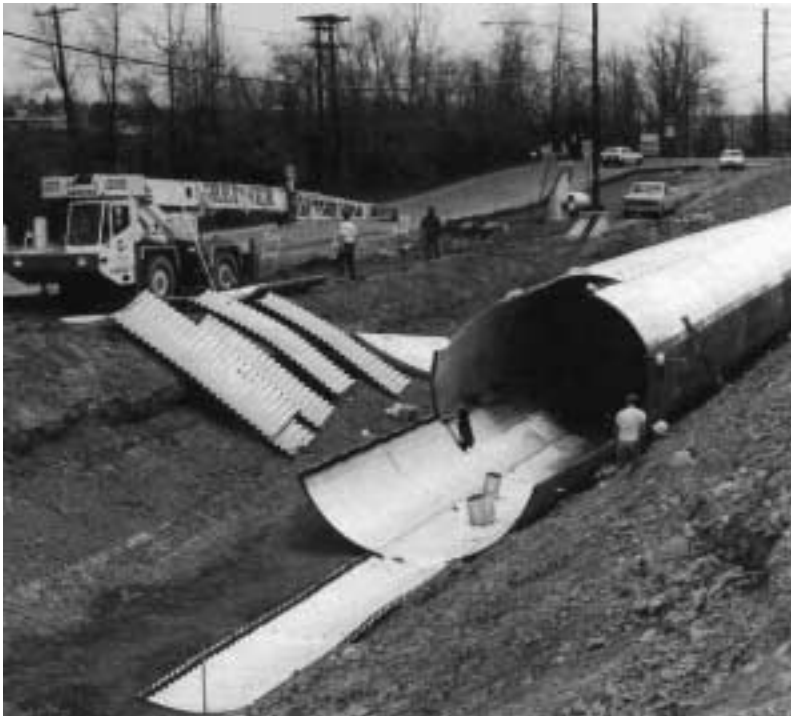
100 m (320 ft) of 3825 mm (12 ft - 5 in.) diameter structural plate pipe with gasketed seams used as an underground detention chamber collecting runoff from a shopping center near Harrisburg, PA.
