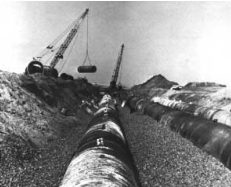
Large storm drain projects under runways at a major airport.
