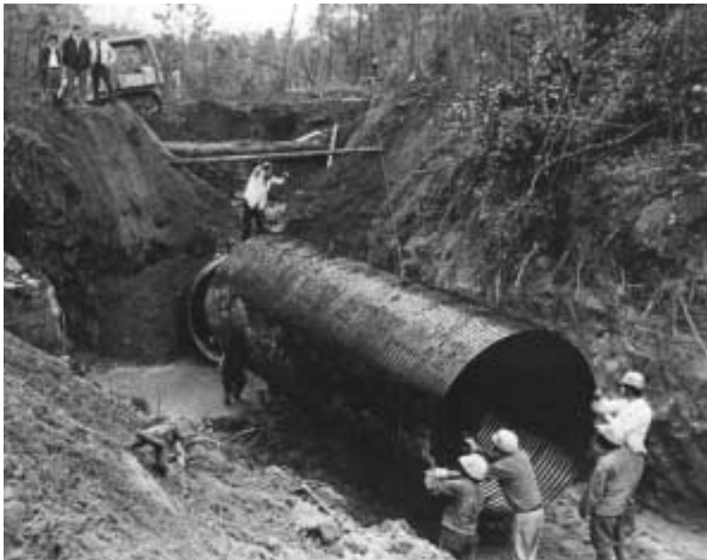
Speed and ease of installation is a major factor in the choice of CSP for storm drainage.
