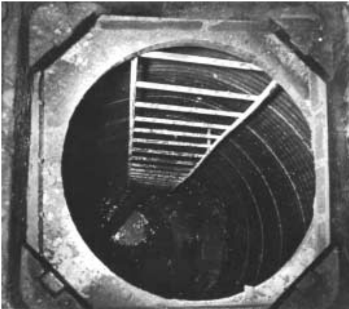
CSP catch basin with concrete slab and standard cast-iron frame and cover.
