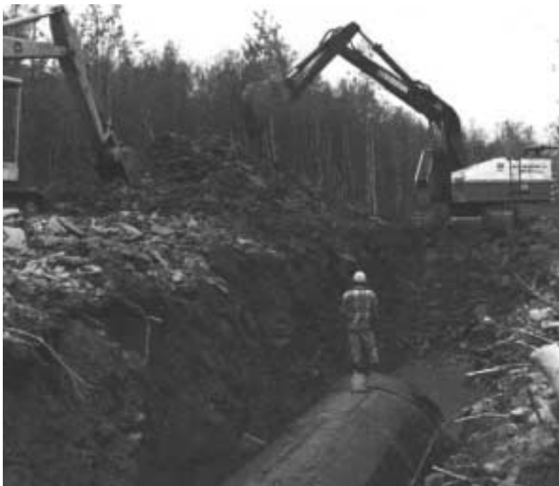
Quick installation of CSP sewer keeps pace with modern trenching equipment.
