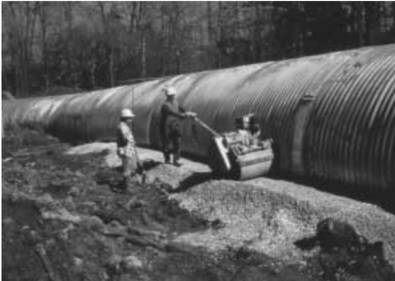
Compacting backfill is required for proper installation of all sewers.
