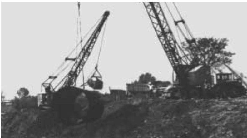
CSP is easy to install in difficult trench conditions.
