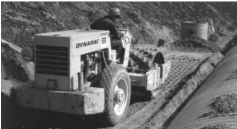
Proper installation techniques are always important.
