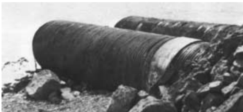
Twin outfall lines for major urban storm sewer system.
