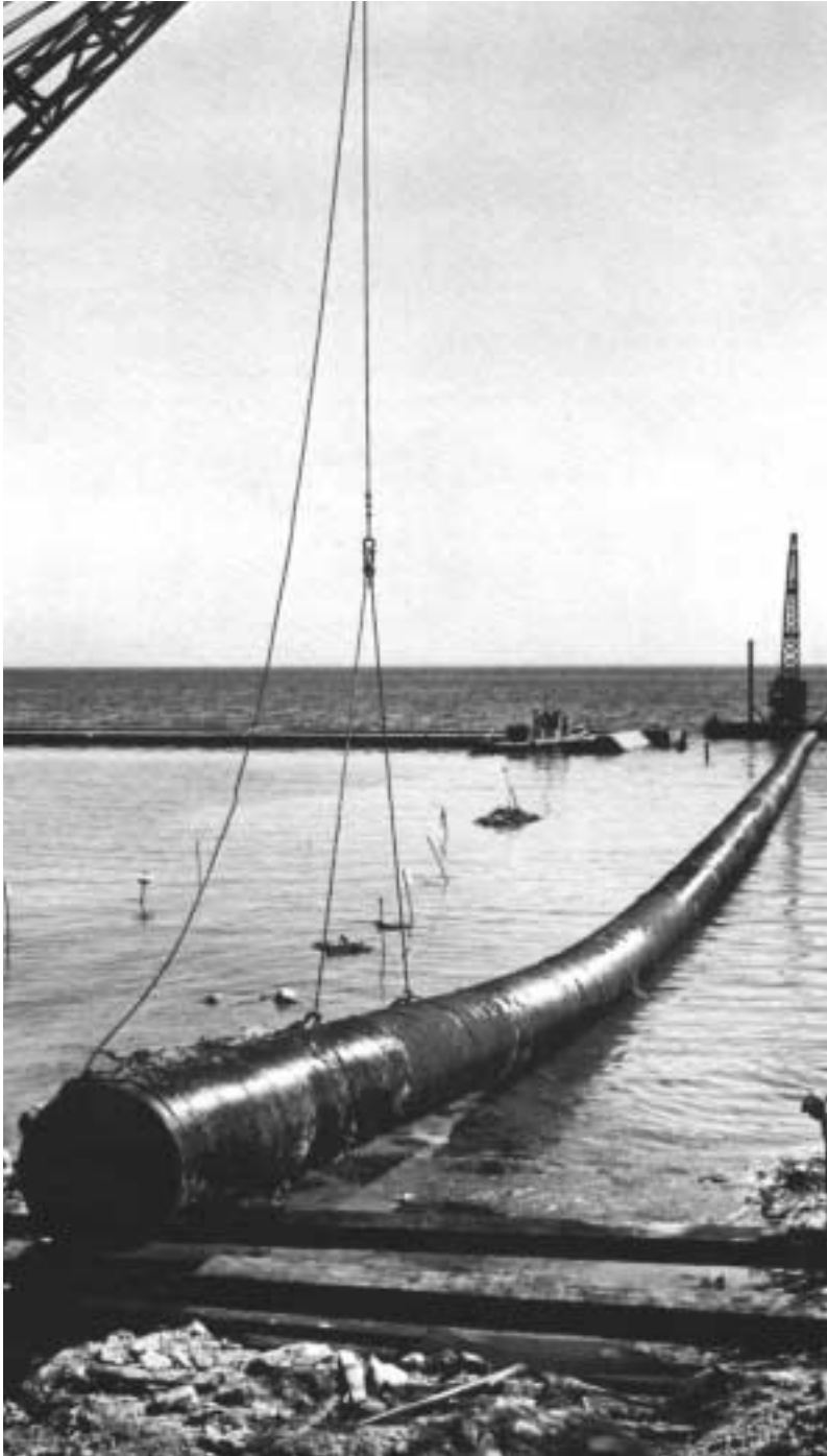
Installing subaqueous corrugated steel sewer pipe.
