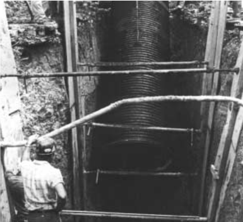
Full bituminous coated and full paved, 75 mm x 25 mm (3 x 1 in.) corrugation, approximately 940 m (3100 ft) of 300-1800 mm (12 - 66 in.) for storm sewer.
