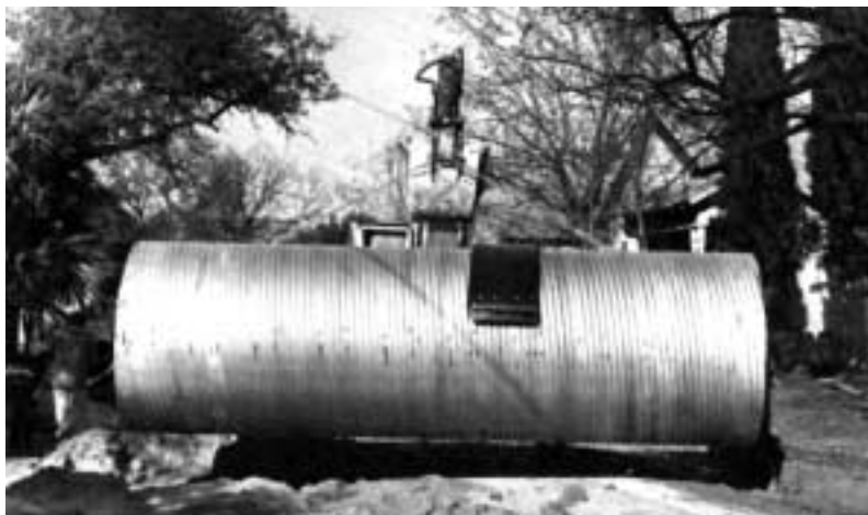
Installing a fully paved sanitary sewer.
