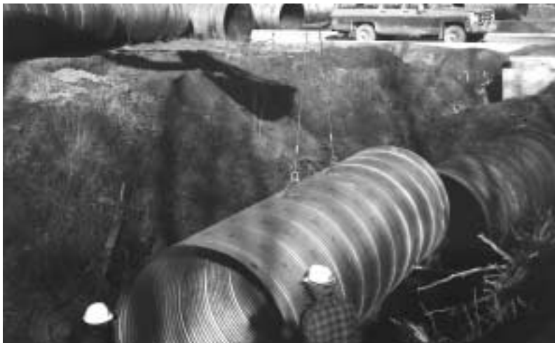
Lifting lugs are provided to protect the exterior coating on this CSP.
