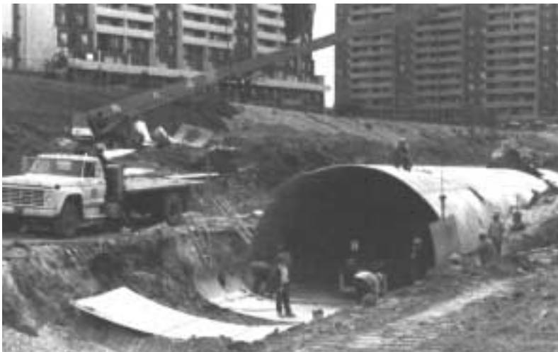
Structural plate storm sewer encloses stream in an urban area.
