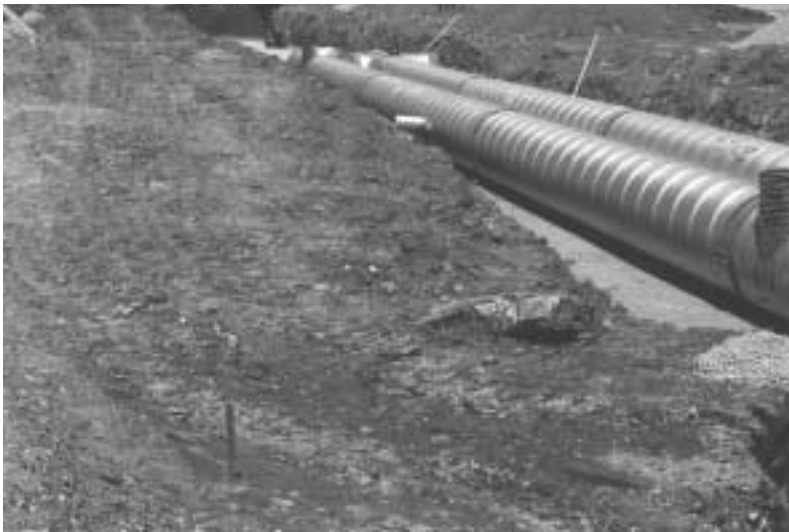
A twin run of 1200 mm (48 in.) diameter CSP provide an underground stormwater detention system for a site.
