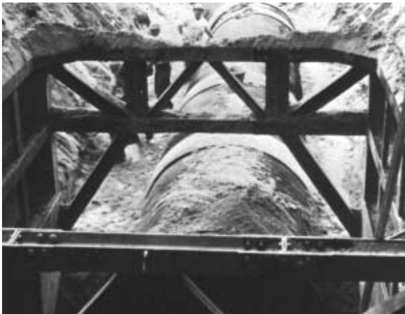
Using steel trench shield to install CSP sewer.
