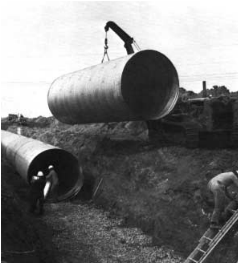
Long lengths with fewer joints can lower the effective “n” value.
