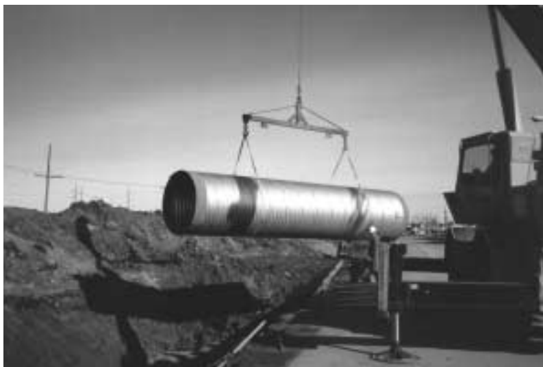
Exterior coatings are protected during installation by use of lifting lugs or slings.
