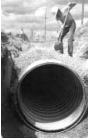
Spiral rib pipe installation.
