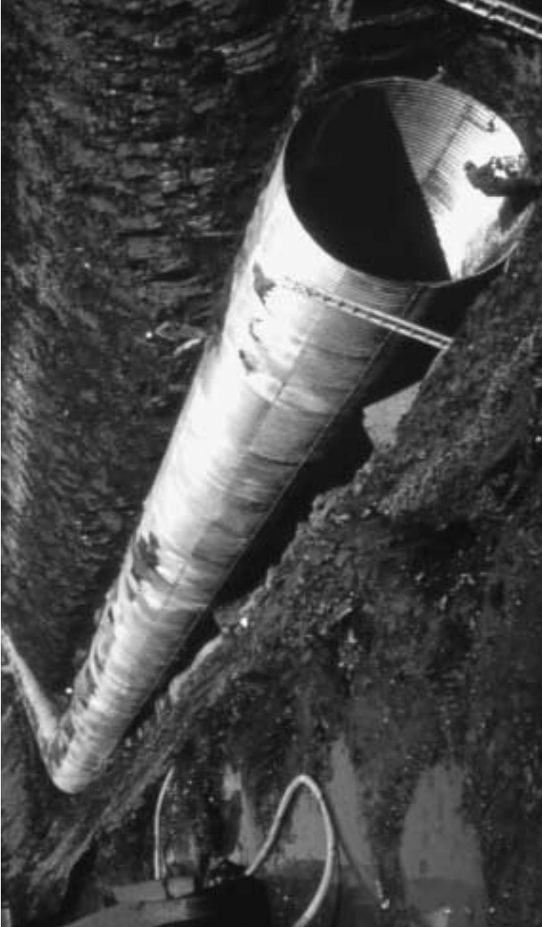
7 m (24 ft) diameter steel sewer being installed in wet conditions.
