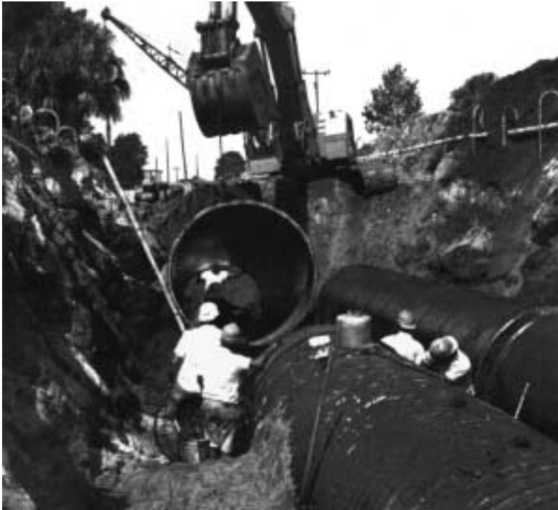
Smooth-lined CSP storm sewer being installed.
