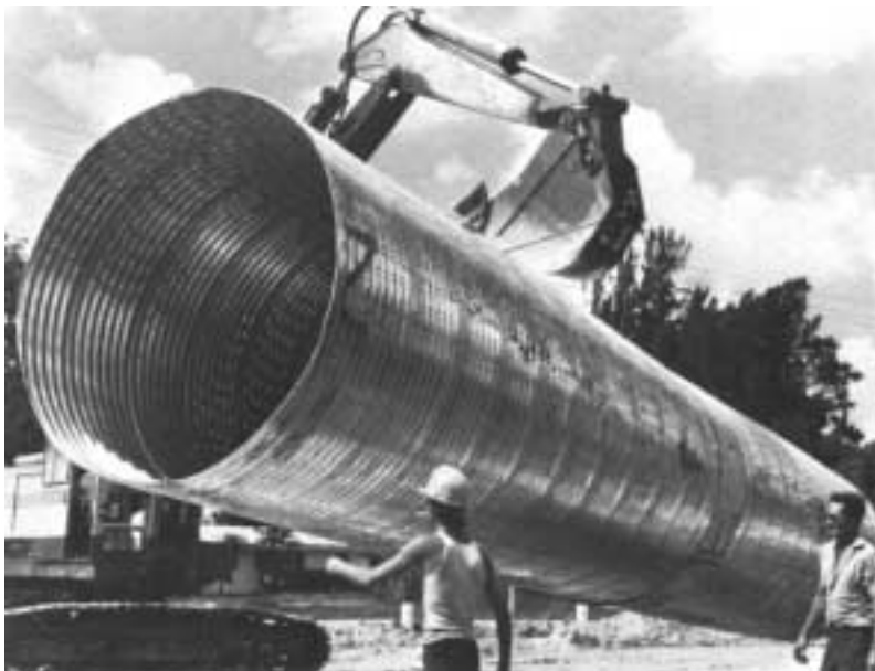
12 m (40 ft) length of 2100 mm (84 in.) fully perforated pipe banded together for installation.
