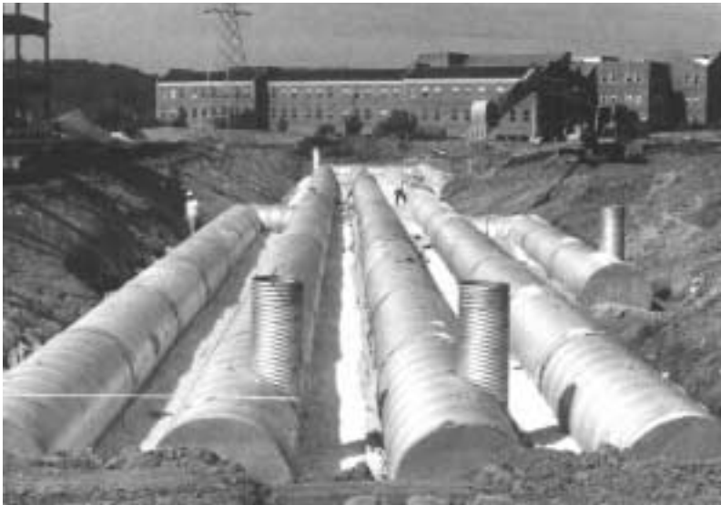
An example of a combination underground detention chamber and recharge system. Five lines of 1800 mm (72 in.) diameter corrugated steel pipe with 150 mm (6 in.) slots in the invert.
