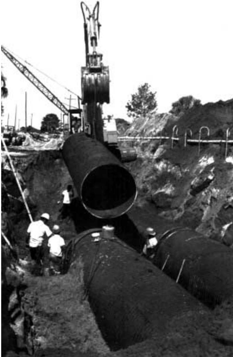
Well points and wide trenches were necessary to install full-bituminous coated and full-paved CSP in this unstable ground.
