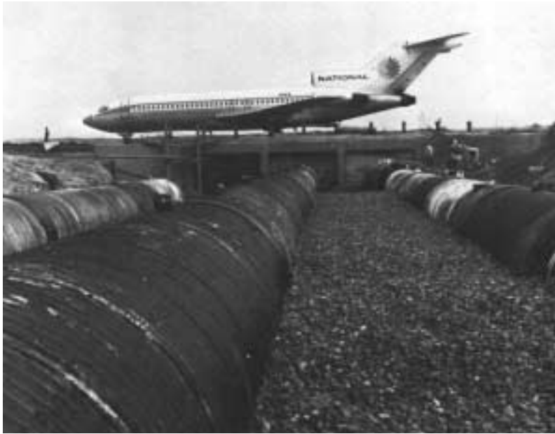
CSP was a cost effective solution for the Newark Airport.
