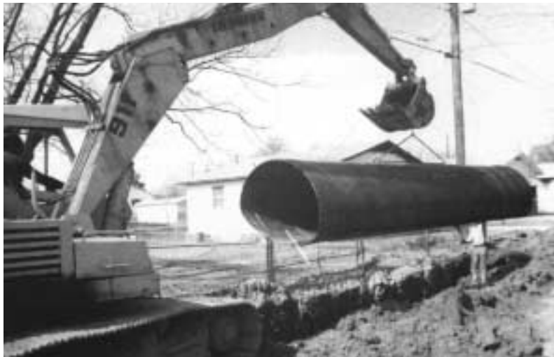
Lengths of pipe-arch are easily moved into position.
