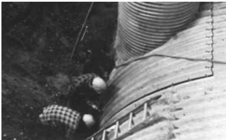
Saddle branch manhole is bolted in place.
