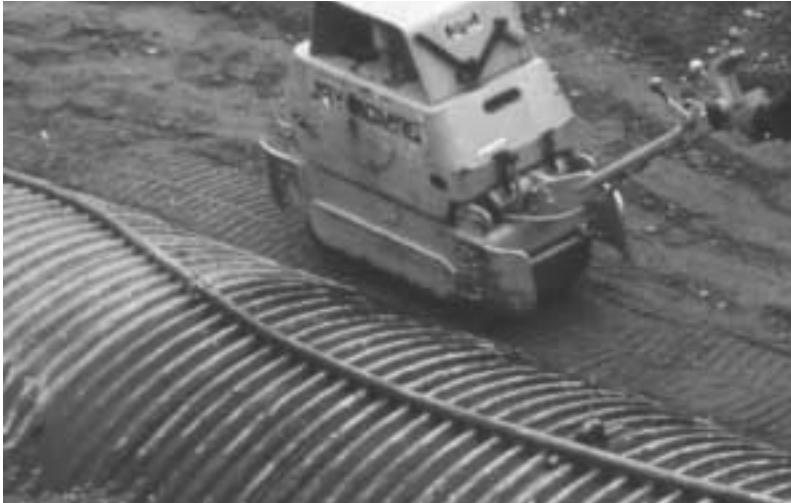
Adequate, uniform compaction is the secret to building soil and steel structures.
