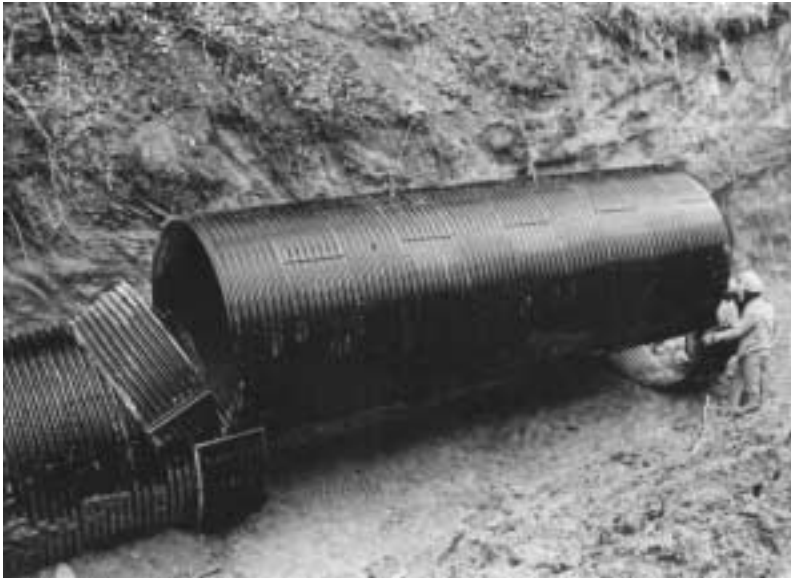
Long lengths and simple mechanical joints are two of the cost saving features of CSP.
