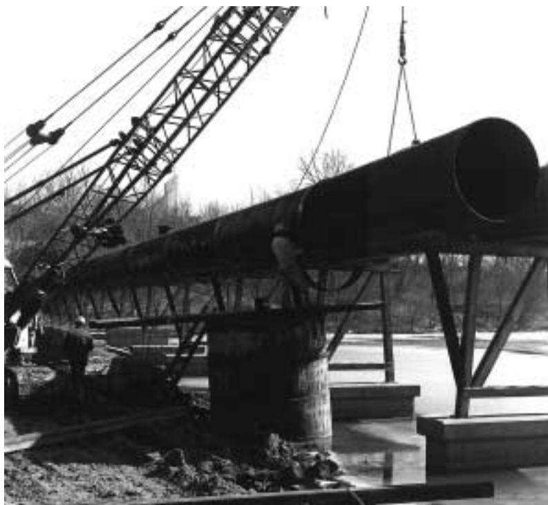
CSP aerial sewer being installed.
