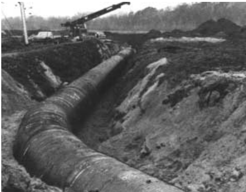
Installation of CSP sanitary sewers.
