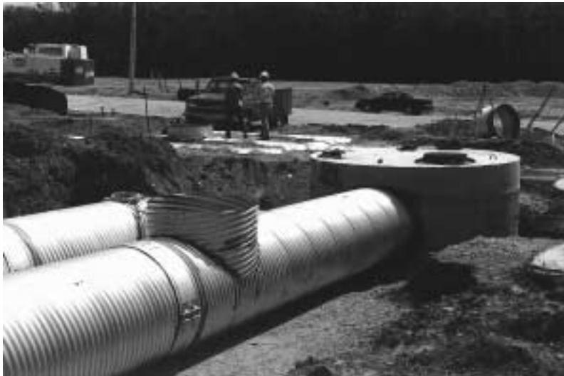
Recharge trench installation showing junction box.
